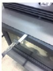
Bypass located above door
